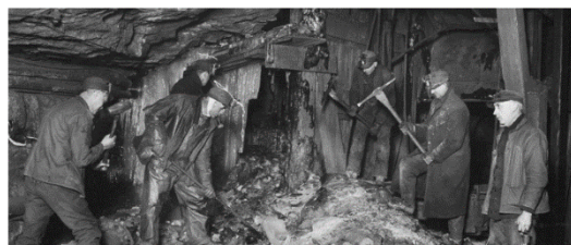
McIntyre Powder Project
